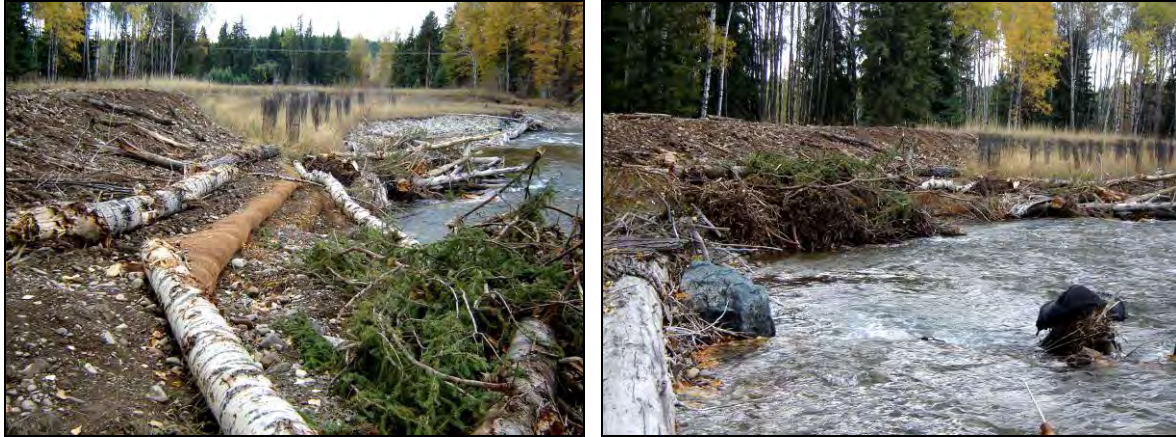
Figure 27. Woody debris jams constructed at Site 10 to reduce bank erosion at the site and allow willow cuttings in the soil lift establish.
