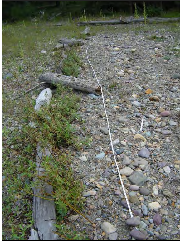
Figure 41. Photograph showing buried coir/willow fascine at Site 13. Effectiveness monitoring data were collected in five-foot increments along each structure.
