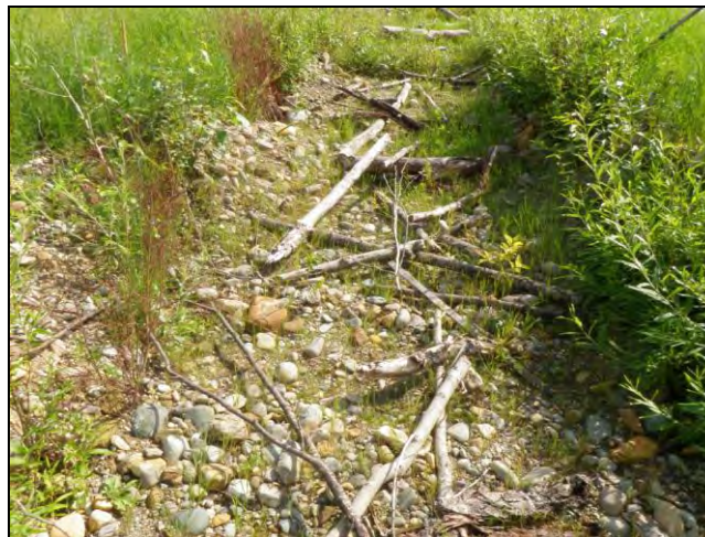
Figure 47. Photograph showing the downstream portion of the vegetated set back bank treatment. Willow growth along the side closest to the channel is dense and seeded grasses are establishing on the bottom of the trench.
