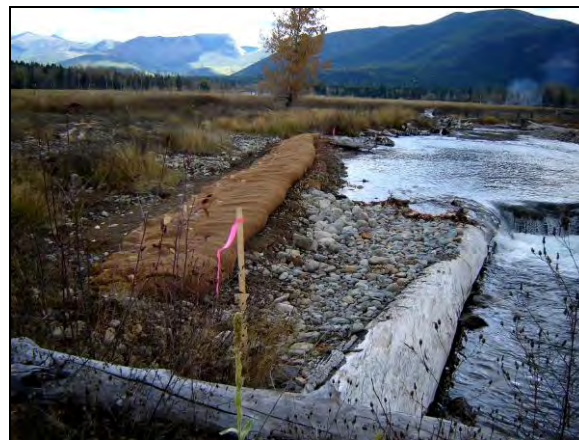
Figure 26. Vane at Site 7 after repairs showing the filled vane arm and reconstruction of the bank line along the decommissioned cattle water gap.
