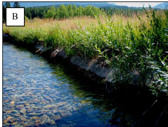
Figure 4. Photograph A shows soil lift 2 constructed in 2006 with a log and rock toe. Photograph B shows soil lift 4 constructed in 2005 without only a cobble toe. Soil lift 4 has more than 80% toe scour and soil lift 2 has 0% toe scour. Willow survival is high on both vegetated soil lifts. Willows growing in the top layer of both lifts had signs of browse.
