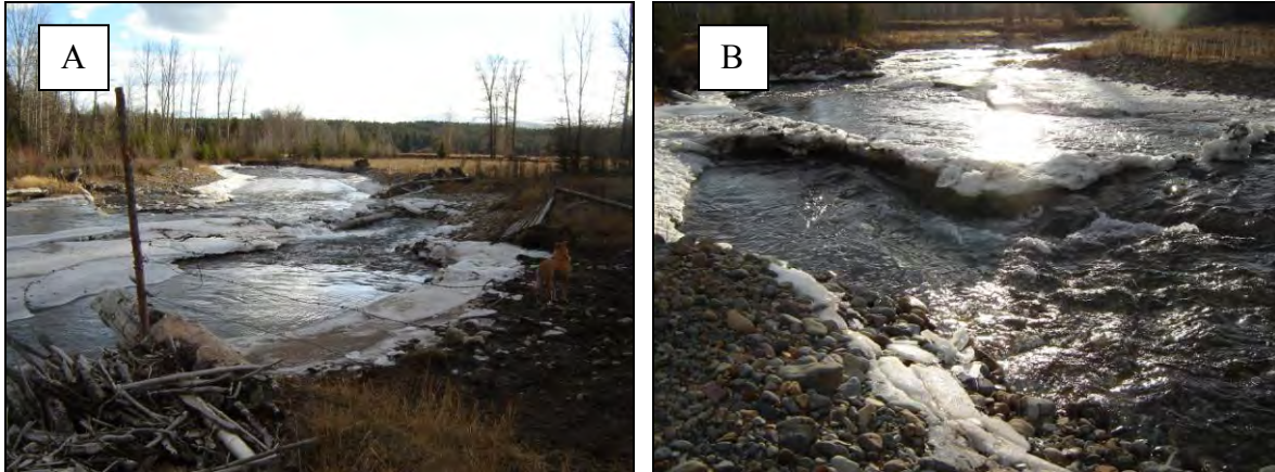
Figure 8. Photograph A shows the structure at Site 7 requiring repairs due to flanking behind the structure arm resulting in accelerated lateral bank erosion. Photograph B shows the structure at Site 8 requiring repairs also due to flanking behind the structure arm.
