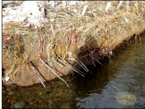
Figure 3. Photograph showing vegetated soil lift installed in 2005 with new willow shoot growth near the base of the stems.
