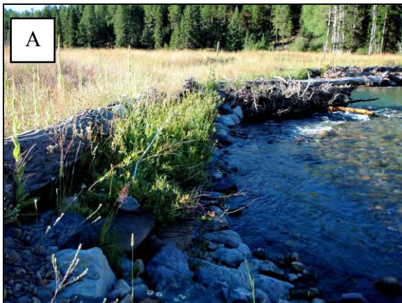
Figure 4. Photograph A shows soil lift 2 constructed in 2006 with a log and rock toe. Photograph B shows soil lift 4 constructed in 2005 without only a cobble toe. Soil lift 4 has more than 80% toe scour and soil lift 2 has 0% toe scour. Willow survival is high on both vegetated soil lifts. Willows growing in the top layer of both lifts had signs of browse.
