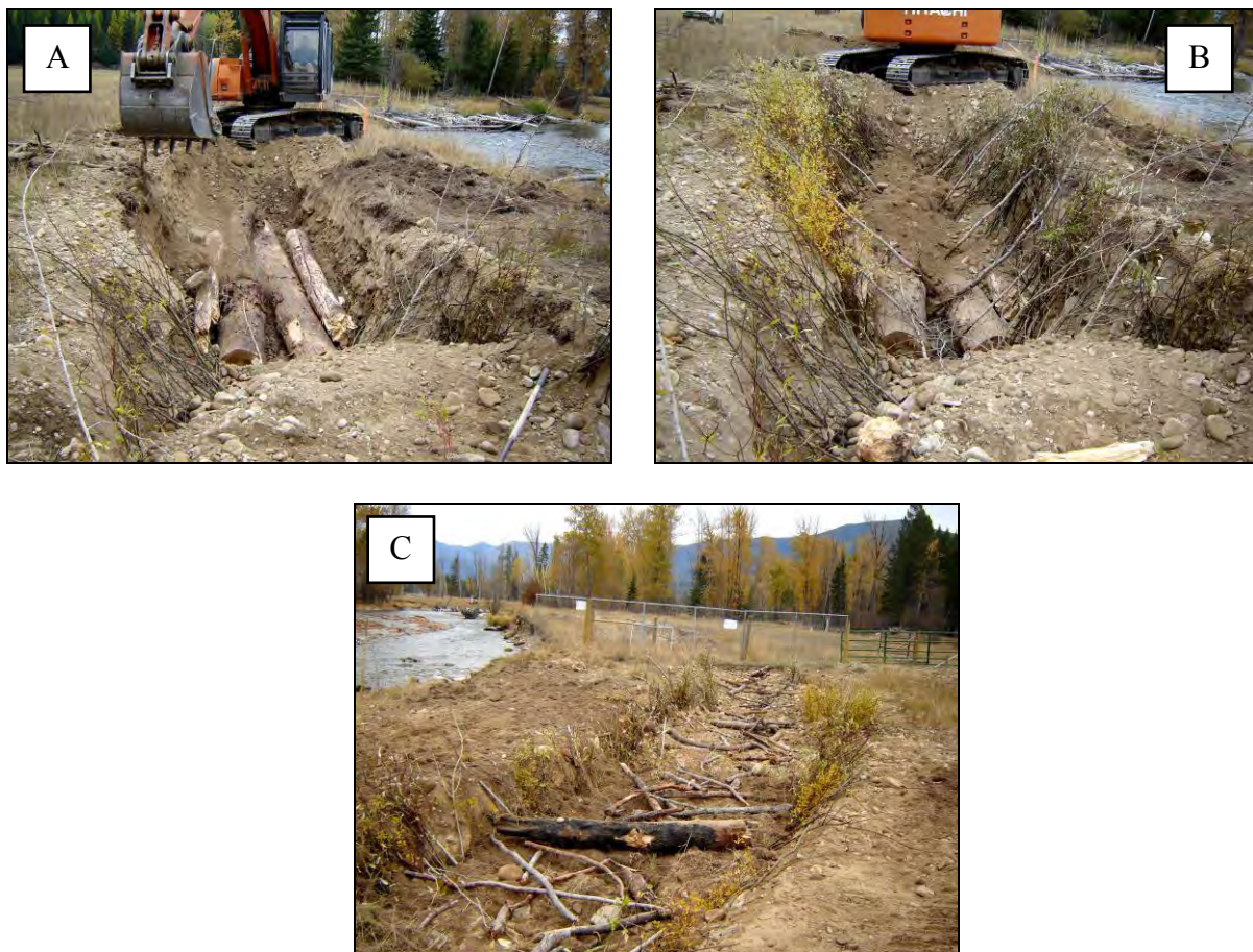
Figure 25. Photographs A through C show the sequence of constructing the vegetated set back bank at Site 2. The trench is excavated to the desired depth, woody debris is placed in the bottom of the trench for structure (Photograph A) and dormant and live plants placed in the trench (Photograph B). The trench is then back-filled to approximately bankfull elevation of the existing channel and container plants are installed and woody debris and seed scattered on the top surface (Photograph C).
